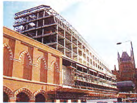
Midland Grand Hotel extension under construction
