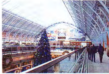
The upper level of The Arcade , looking south under Barlow's roof, just after opening to the public and just prior to Christmas 2007
